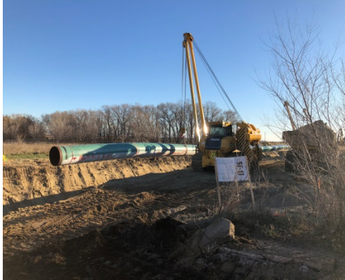
SF 8, oak creek crossing, photo facing north east, pipe being lowered into the trench.
