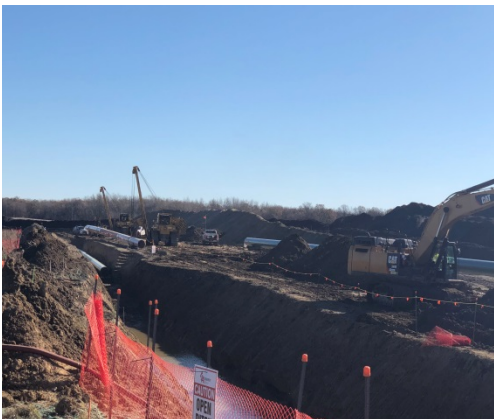
SF 38, photo facing south east, excavator moving soil, side booms moving pipe closer to trench.
