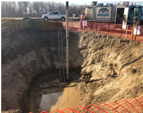
SF 38, hydro vac pumping out water from open ditch, you can also see the boring drill bit just above the water.
