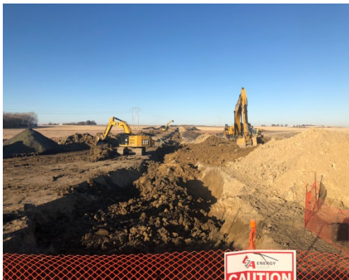
SF 30, photo facing east, backfilling taking place.
