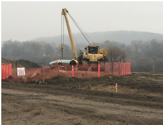
SF 35, photo facing south east, side boom raised pipe and crew members built up skid pile higher.
