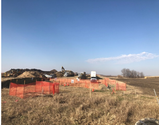
SF 38, photo facing north west, boring taking place.
