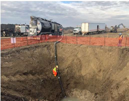
SF 41A, photo facing west, hydro vac pumping out water while directional drill drills.
