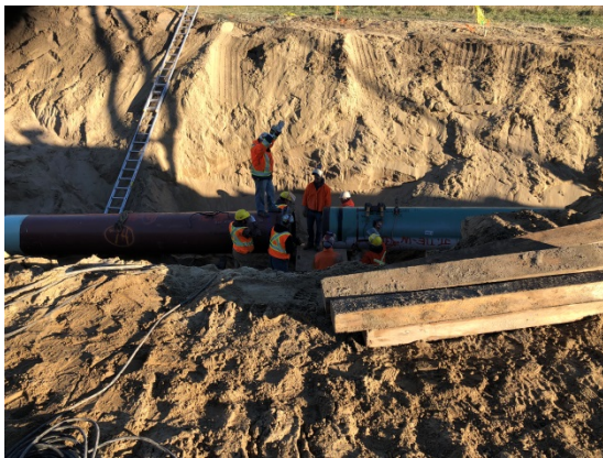
SF 8, oak creek crossing, one crew member giving signals to the boom operators to line the pipe up with the pipe that's already in the trench.
