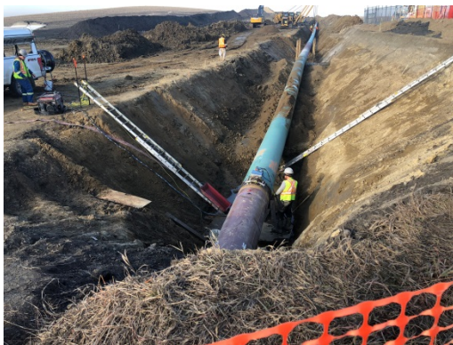
SF 28, photo facing west, lowering in crew lowering in pipe, APPlus doing ultra sounds on the pipe.
