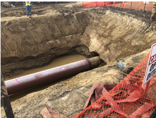
SF 38, photo facing west, pipe is under the road being pulled by the directional driller.
