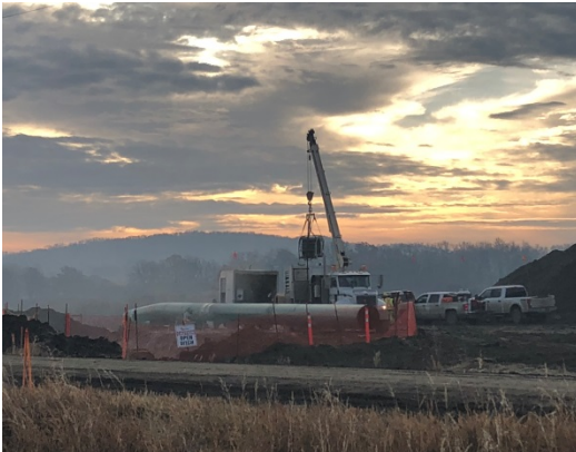
SF 35, photo facing south east, sand blasters sand blasting the pipe, coaters came shortly after.
