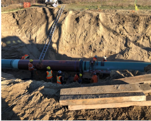
SF 8, oak creek, pipe lined up, two crew members heating up the pipe with tiger torches to prepare for the welding.
