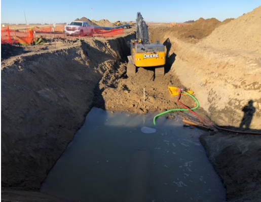
SF 35, photo facing west, excavator moving out dirt, crews attempting to pump out water.
