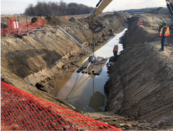
SF 38, photo facing south east, a picture of the drill bit that was used to boar under the road with the pipe attached.
