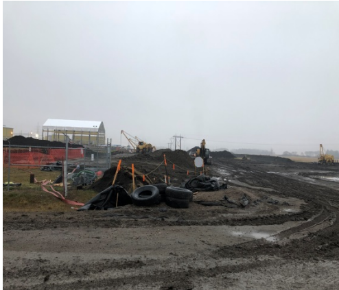
SF 20, photo facing east, lowering in crew lowering in pipe, ROW is very muddy and wet.
