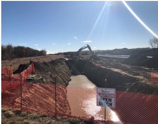
SF 38, photo facing east, excavator digging dirt out of trench, one dozer pushing that dirt to the side of the row. Lots of water in the trench.
