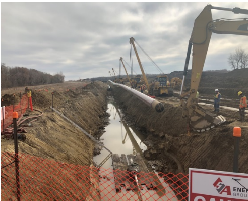
SF 38, photo facing south, lowering in crew getting ready to lower in pipe and attach it to the drill bit.
