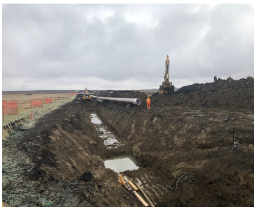
SF 43, photo facing east, excavators moving dirt out of the trench to the side of the ROW.
