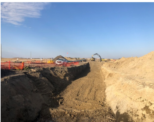
SF 35, photo facing west, excavator loading dirt from the trench into the back of a rock truck.
