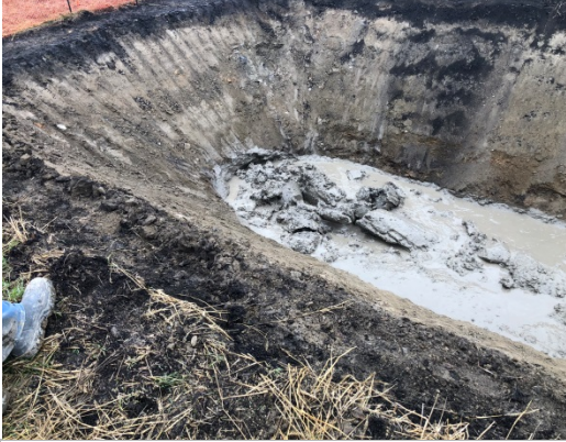
SF 41A, photo facing north west, drill bit coming out on the east side of the road.
